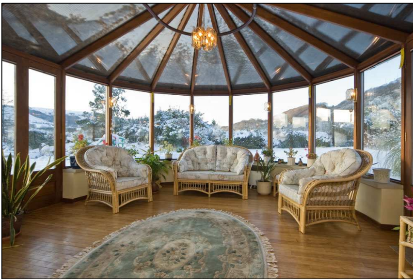
CONSERVATORY (5.0mx4.2m) constructed from 'Iroko' hardwood, double glazed and with the benefit of 'Sanderson' blinds and two pairs of external doors to patio and garden. Bronze tint polycarbonate roof with 4no automatic roof vents and a solid hardwood floor.
